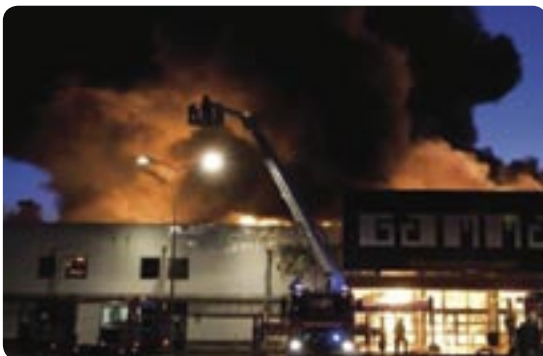
Insulation material type is not the most important factor, e.g. 2008 fire at a Gamma DIY store (NL) with non-combustible insulation.
